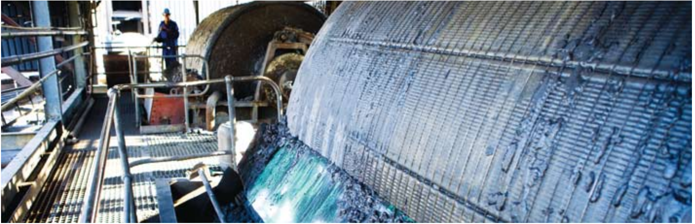
Consolidated Murchison: Flotation plant
