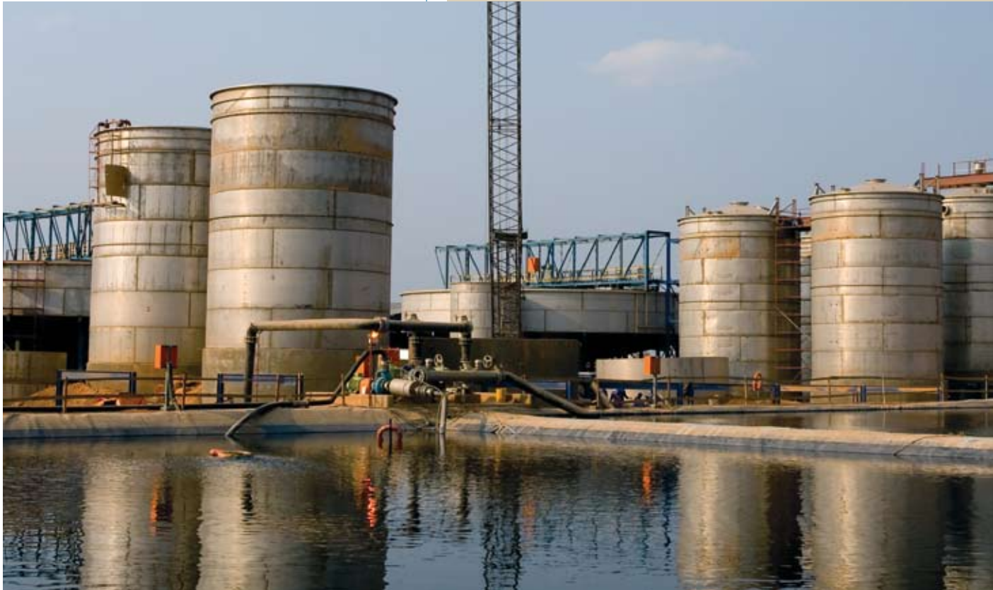
CCD tanks (Ruashi view over PLS pond)
